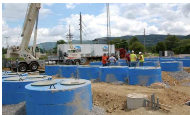
Volant fibre carbone 1 tonne 8000 – 16 000 tr/min
